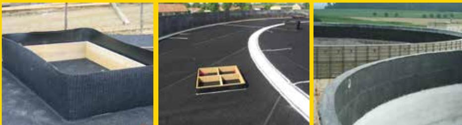
AGROTEL WireTarp concrete protection film is made of a polypropylene-coated loop fabric. It is easy and convenient to install and weld in the relevant areas. WireTarp is a perfect all-round solution for concrete protection.
