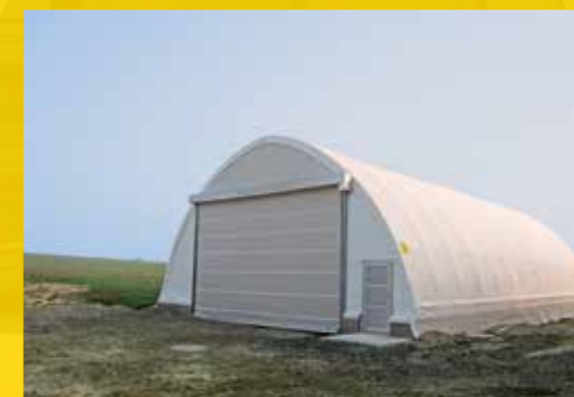
Tunnel Hall with Big-Rib Rollup Door
