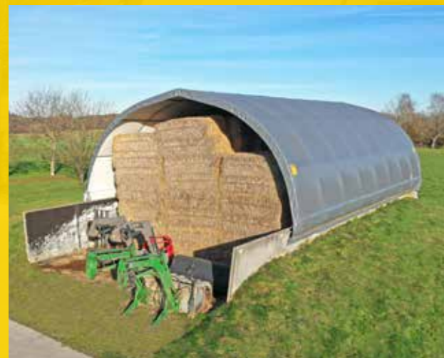
Tunnel Hall construction on bunker silo
